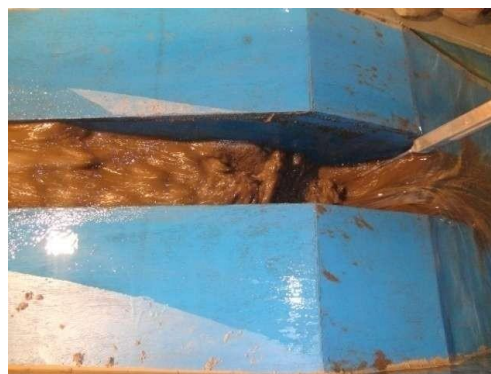
Figure 6 (a): Widening of breach
