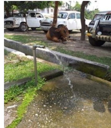
Plate 1: Wasting the Fresh Water at Ukilpara.
