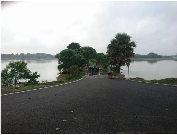
Figure 2: Photograph of flood affected area in Bhojpur district
