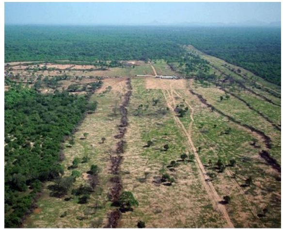
Figure 2: Image of the clearance work of MRIA Runway (Source: www.slpa.lk)
