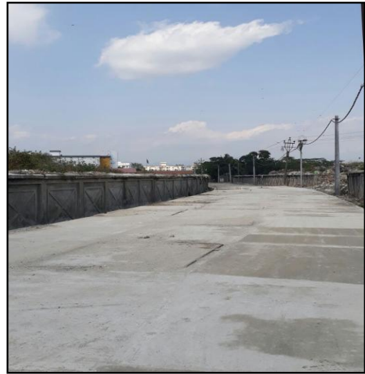
PLATE 5: CONSTRUCTION OF NEW ROAD AROUND DUMPING GROUND
