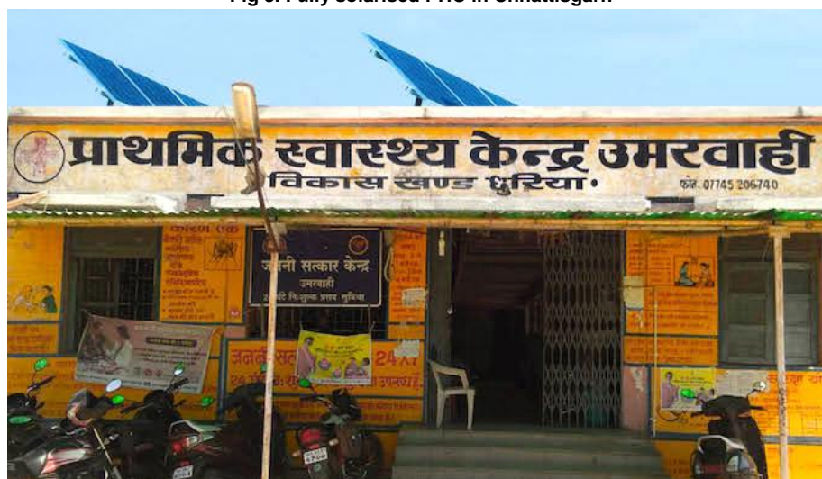
Fig 3. Fully solarised PHC in Chhattisgarh
