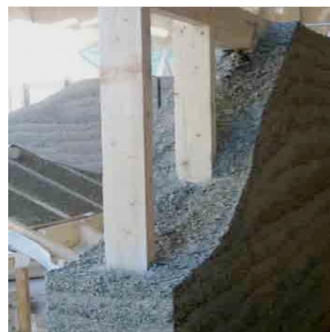
Figure 6 Lime-hemp on a timber frame
