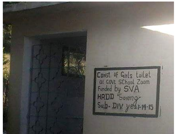
Plate 9: Well prepared modern toilet in school
