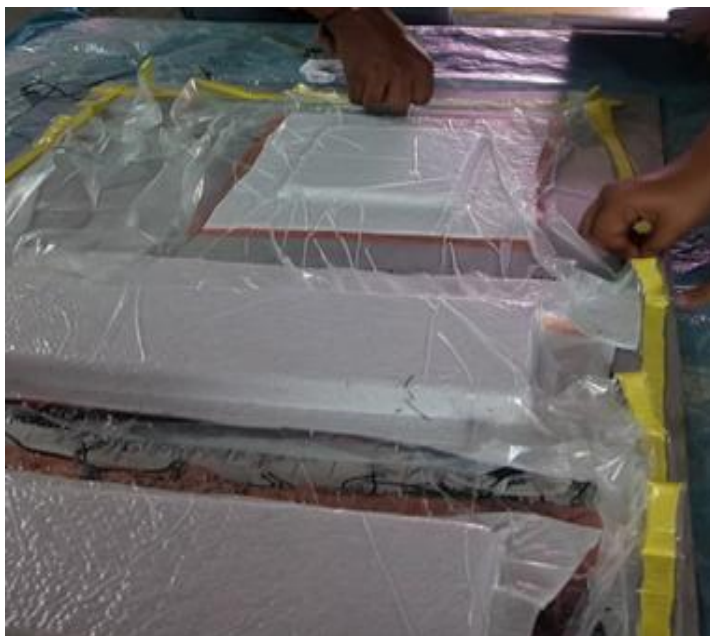
Fig 2. Vacuum Bagging Process
